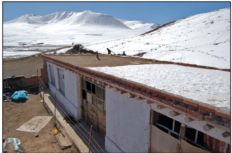
Trial installation of solar-powered electric fencing (SPEF) technology in Lari Village, Zhiduo County, in 2009
